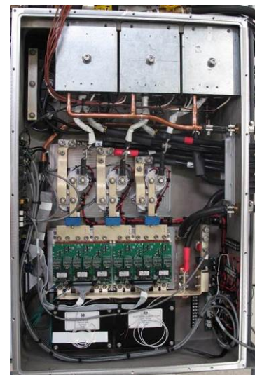
Figure 12. Interior of ICU.
